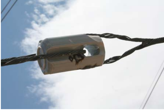
132012071-038 – Jonny Ball Insulator Lower East Guy Wire
