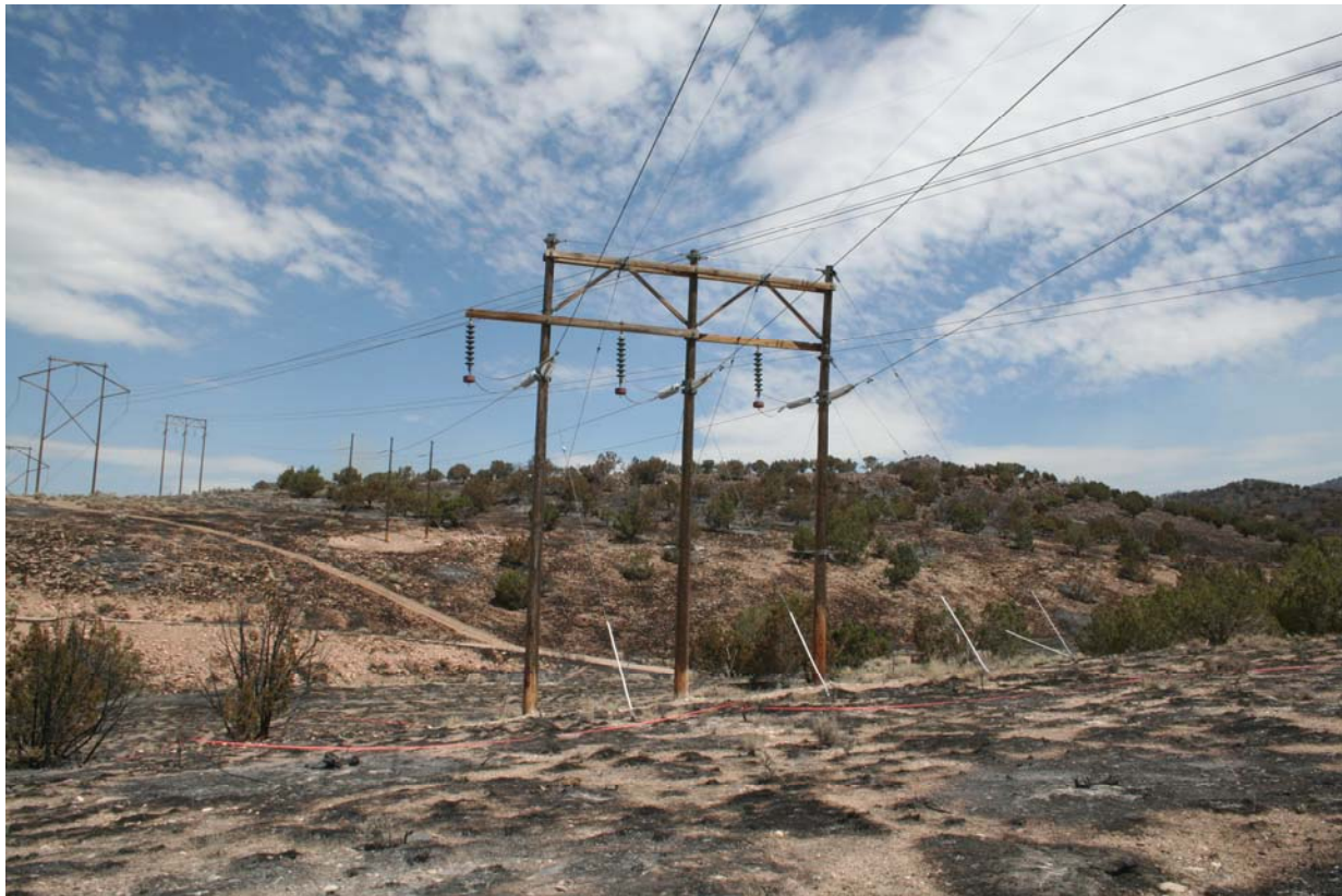
132012071-027 – 138 KV Double Dead End Structure – Looking to the Northeast
