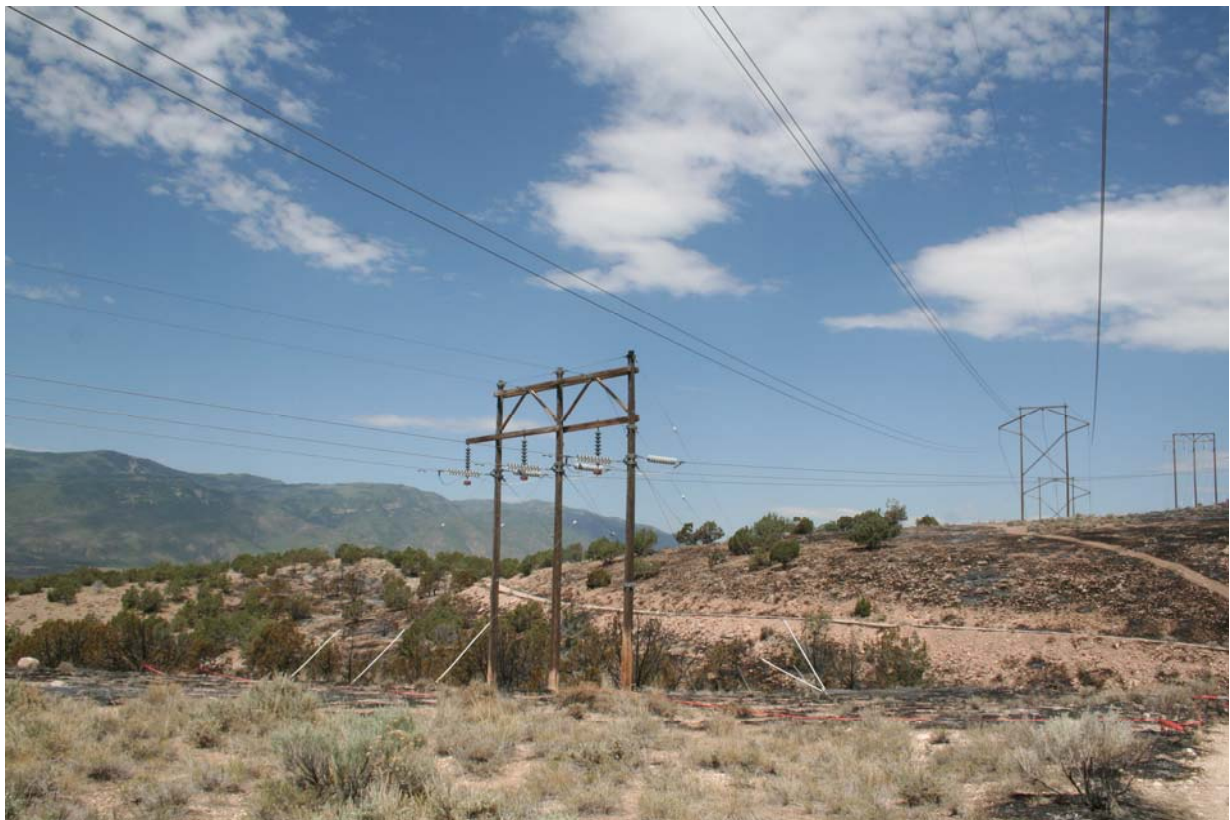
Photo 132012071-024 – 138 KV Double Dead End Structure – Looking to the Northwest
