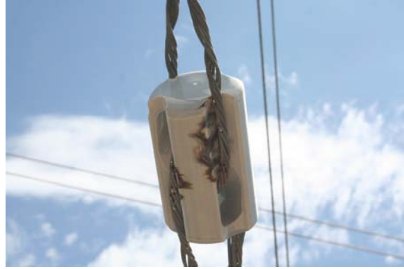
132012071-039 – Jonny Ball Insulator Lower East Guy Wire
